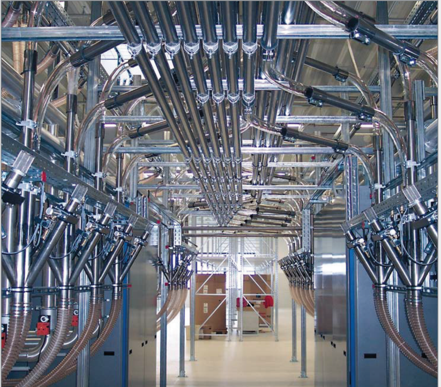
Central conveying system with three CKT dryers and 30 drying containers. The conveying pipes and bends was made in V 2 A (highest-quality stainless steel) and special shatterproof glass. The glass pipes and bends are used for the transport of hard materials and materials containing fibreglass.
