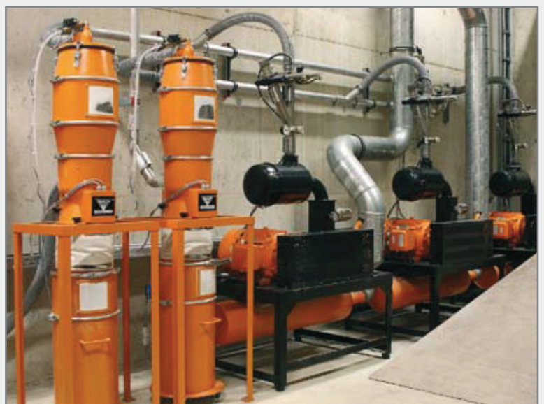
11 kW vacuum pumps and Sa 3 safety filter with 60l collecting tank
